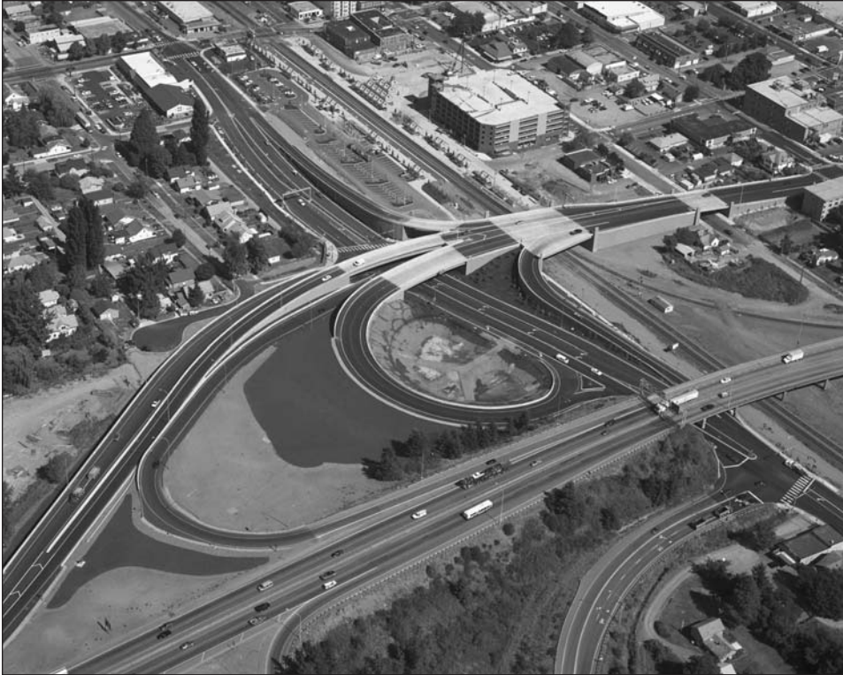
Charles A. Booth Bridge in Auburn, part of FAST Corridor rail and highway project (courtesy of Harris & Associates and City of Auburn)
